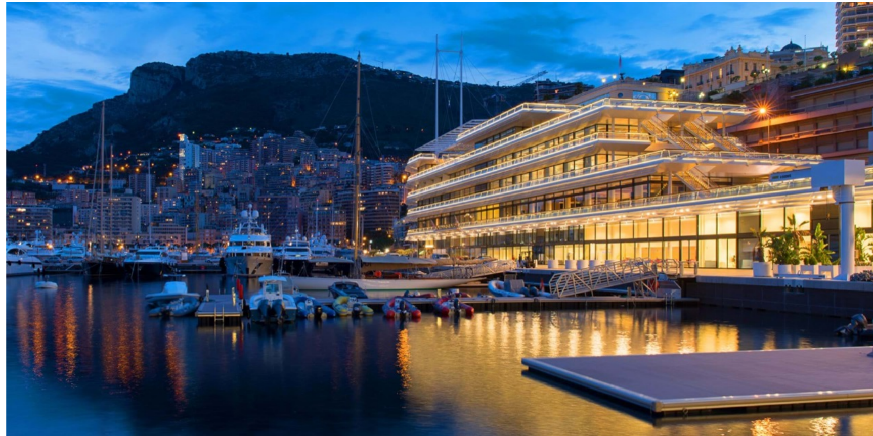
LITERAL FORM PERMANENTLY INSTALLED AT PRINCE ALBERT OF MONACO'S NEW YACHT CLUB DESIGNED BY NORMAN FOSTER.
